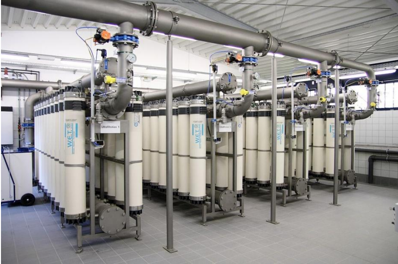
Figure 5.12 – Ultrafiltration designs
