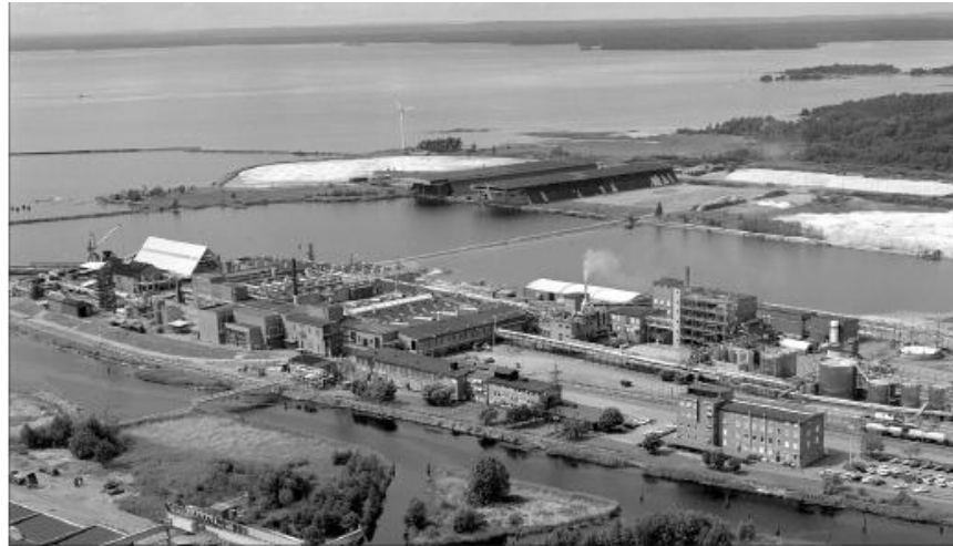
Figure 1.5 - Changing technology. The chlor-alkali factory outside Skoghall in west Sweden once used the mercury electrode method to produce chlorine. In 1987 the new membrane-based technology was introduced, replacing all use of mercury. There has been a 100% change to this new technology in Japan, a partial change in Western Europe and USA, but no change has yet taken place in eastern and central Europe
