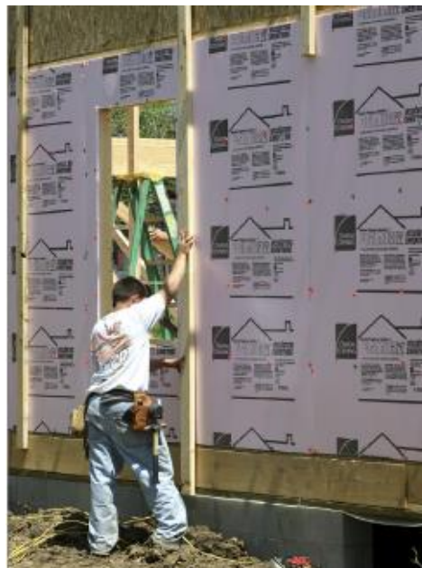
Figure 1.9 - Housing. Insulation of a house as here may decrease energy demands considerably. Additional possibilities for reducing energy costs are installation of a heat pump, and use of solar panels.
