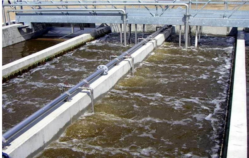
Figure 5.6 -Aerotanks
