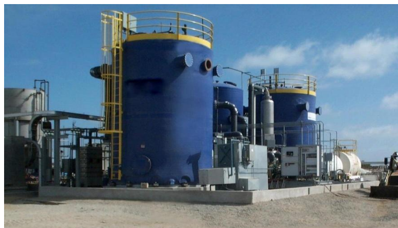
Figure 5.9 - Fluidized bed reactor system
