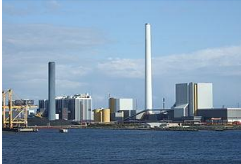
Figure 1.2 - View of Kalundborg Eco-industrial Park
